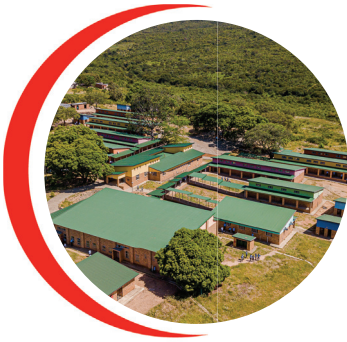
Upgrade to Mathibela High School
