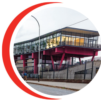
New Westbury Transformation Development Centre
