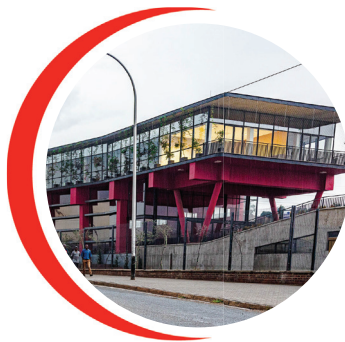
New Westbury Transformation Development Centre
