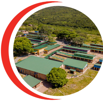
Upgrade to Mathibela High School
