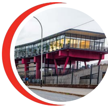
New Westbury Transformation Development Centre
