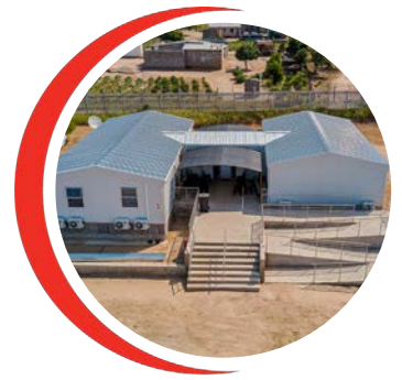
Upgrades to Makoko Clinic
