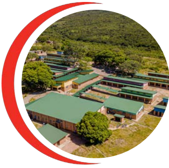
Upgrade to Mathibela High School
